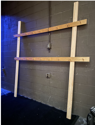
EXAMPLE OF VERTICAL SUPPORT NOTE: VERTICAL SUPPORT STRUCTURE PROVIDED BY VENUE DISCUSS MOUNTING OPTIONS FOR PEG RAIL
