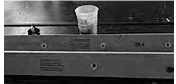
PEG DETAIL SHIPPED LOOSE ATTACHED W/ SHORT DRYWALL SCREW THROUGH BACK OF BOARD
